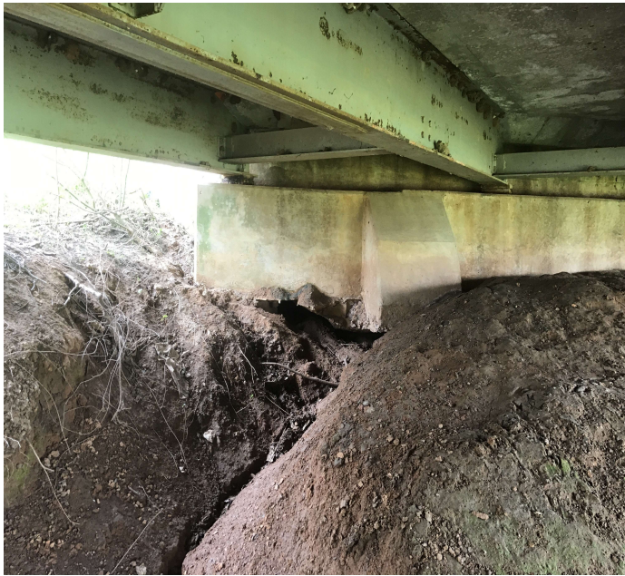
PHOTO 1 Description Bent 8 end slope right has erosion under cap exposing pile1.
