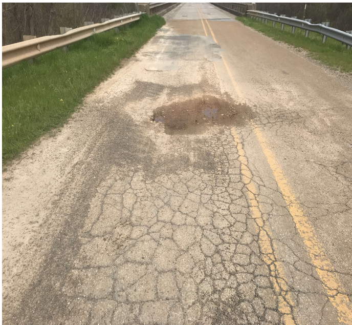
PHOTO 1 Description Approach roadway has potholes and heavy cracking to asphalt.
