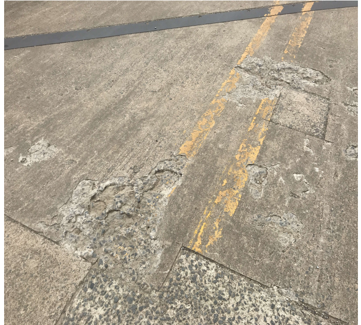
PHOTO 9 Description Deck span 7 has spalls.
