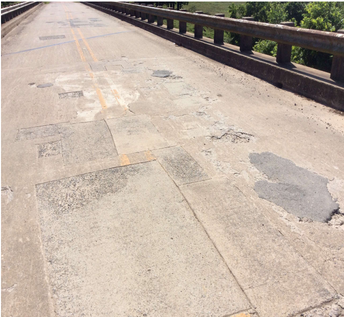
PHOTO 4 Description Deck - Span 3: Spalling
