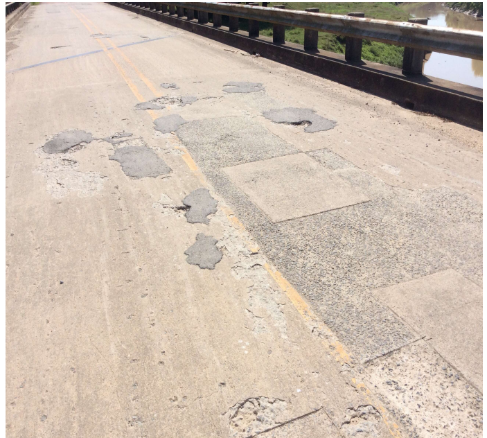
PHOTO 6 Description Deck - Span 4: Spalling
