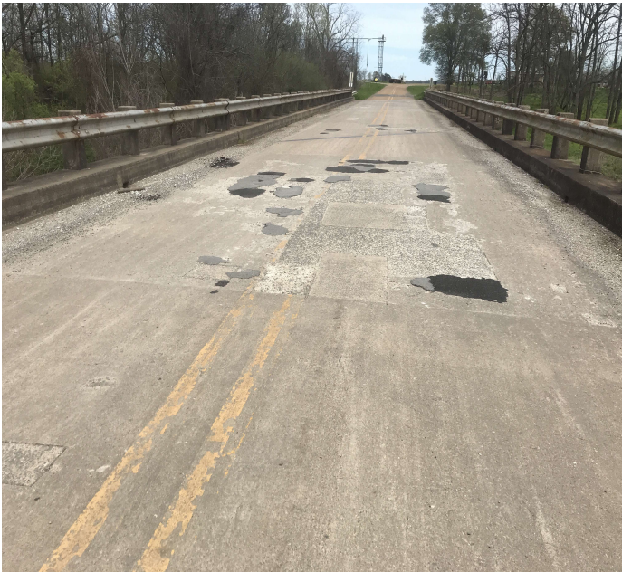
PHOTO 8 Description Deck span 4 many spall delams and patched areas.
