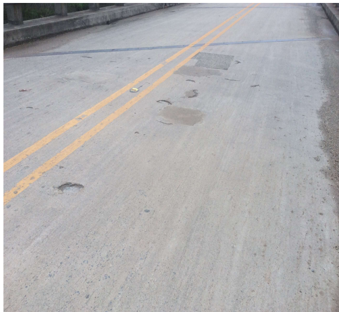
PHOTO 1 Description Span 1 small spalls in deck.
