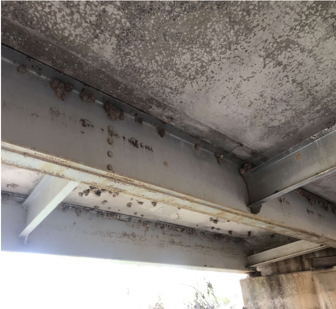
PHOTO 7 Description Typical paint condition of girders.
