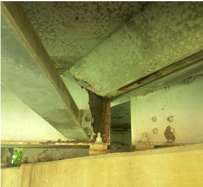
PHOTO 3 Description Span 6 Girder 2 right @ Bent 7: Corrosion
