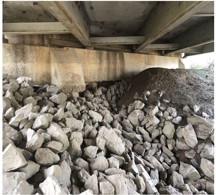
PHOTO 2 Description Bent 1 End slope erosion with rip rap in place.
