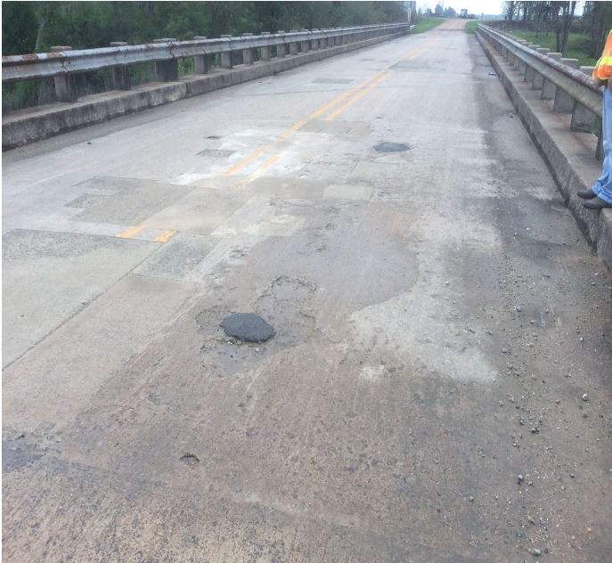
PHOTO 3 Description Span 3 spalls and spalls filled with asphalt.
