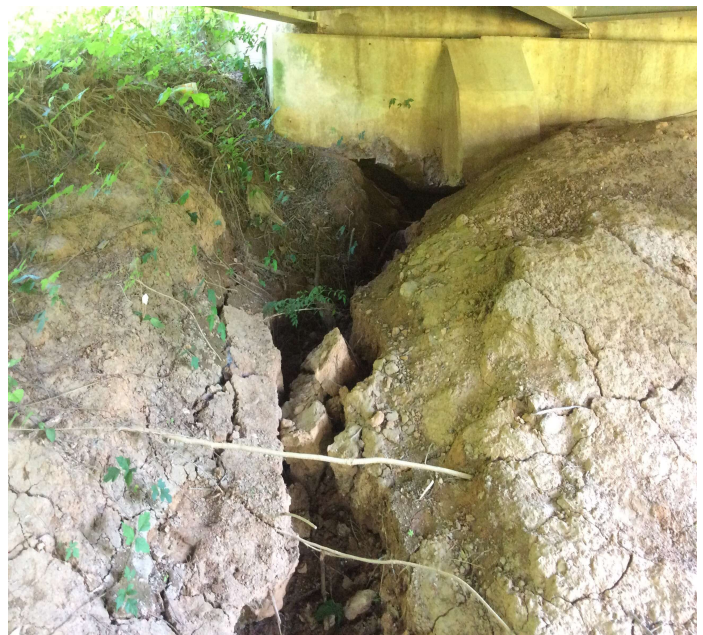
PHOTO 2 Description Endslope - Bent 8: Erosion
