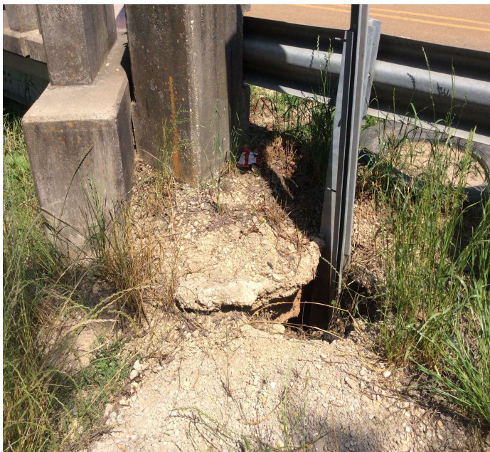
PHOTO 1 Description Approach roadway - Bent 8 right: Erosion
