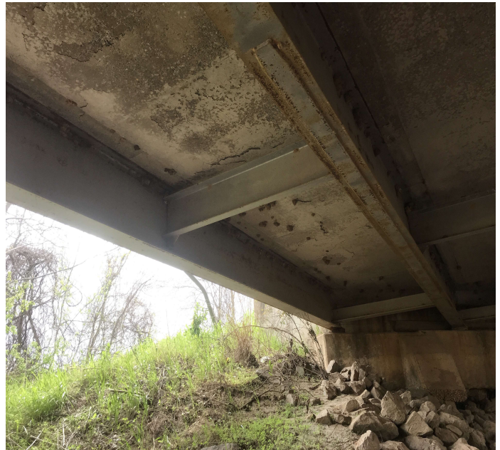
PHOTO 10 Description Span 1 bay 4 has some delams in soffit area. Common bay 1 this span.
