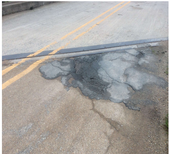
PHOTO 2 Description Approach roadway settlement.
